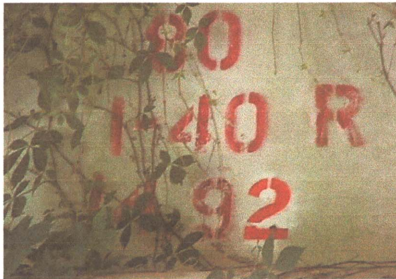
BRIDGE NO. AT ABUTMENT # 1
