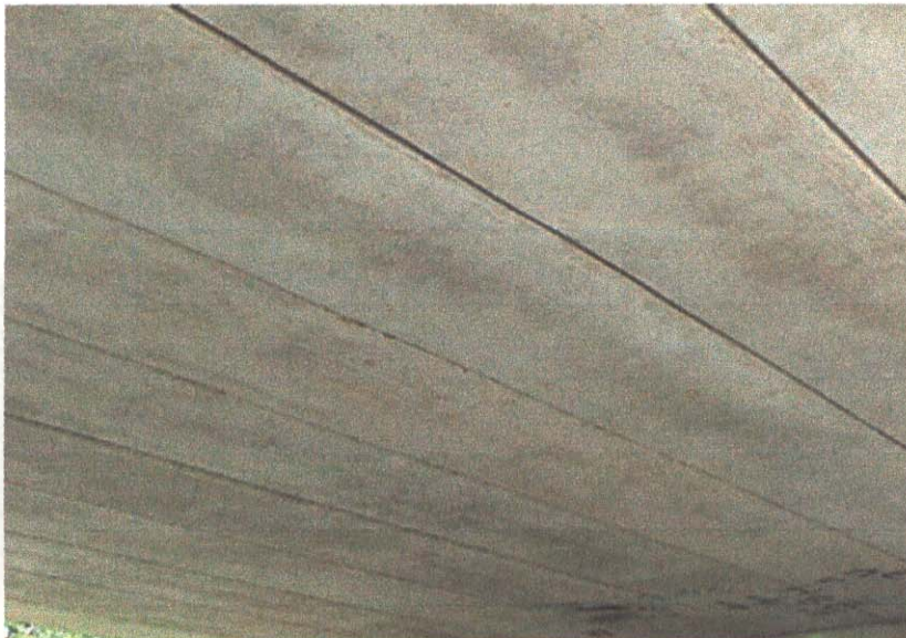
BOTTOM OF DECK
