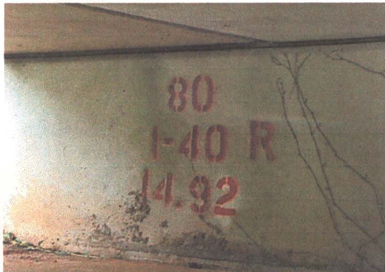
BRIDGE NO. AT ABUTMENT # 1
